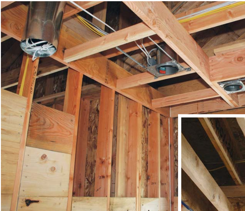
Figure 1. The author uses a single 2x10 fire block nailed to the face of the studs for this kitchen soffit — much faster than installing individual blocks in the stud bays (above). Scraps of OSB rim board isolate a dropped ceiling (right) from the stud cavities on its left and the stair stringers beyond.
