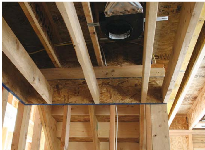
Figure 1. The author uses a single 2x10 fire block nailed to the face of the studs for this kitchen soffit — much faster than installing individual blocks in the stud bays (above). Scraps of OSB rim board isolate a dropped ceiling (right) from the stud cavities on its left and the stair stringers beyond.
