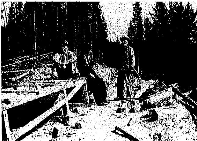
Putting in metal flume. Ted Topham on left.
