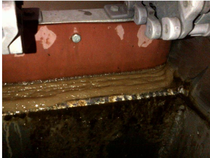
Photo 4.1 – Optimized DAF Float (September 19, 2014)
