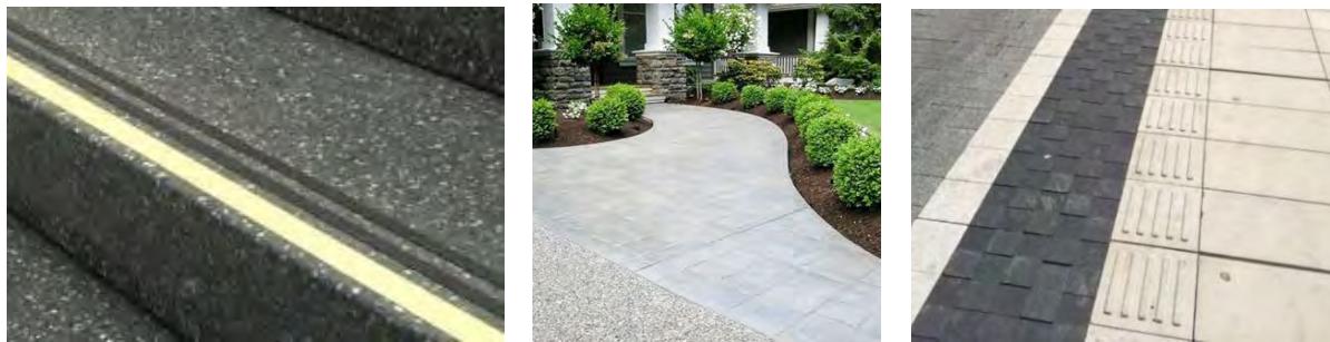
Figure 54: Examples of a colour-contrast, slip-resistant, and tactile surfaces along pedestrian routes to help users move through open spaces.
