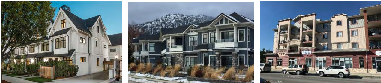
Figure 53: Windows, patios and individual entrances offer passive surveillance and activates frontages.
