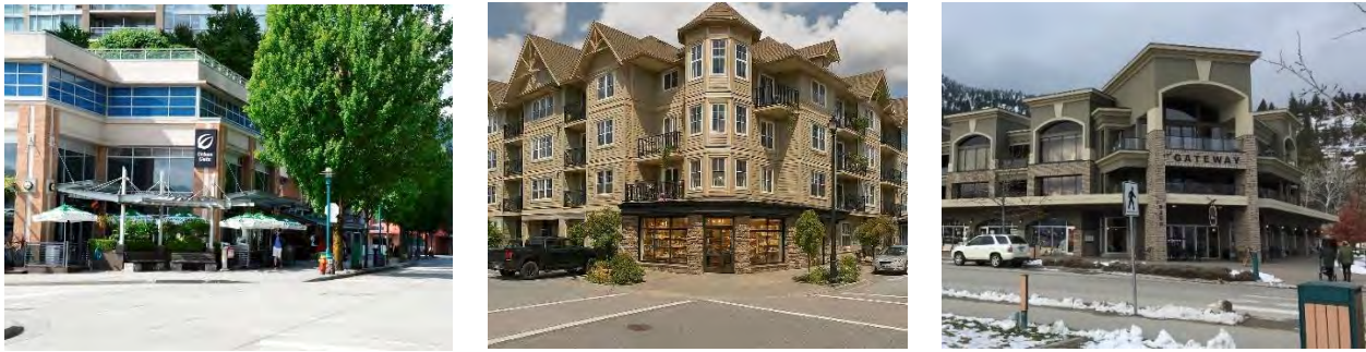
Figure 52: Examples of corner treatments with entrances, balconies and patios that create a focal point.
